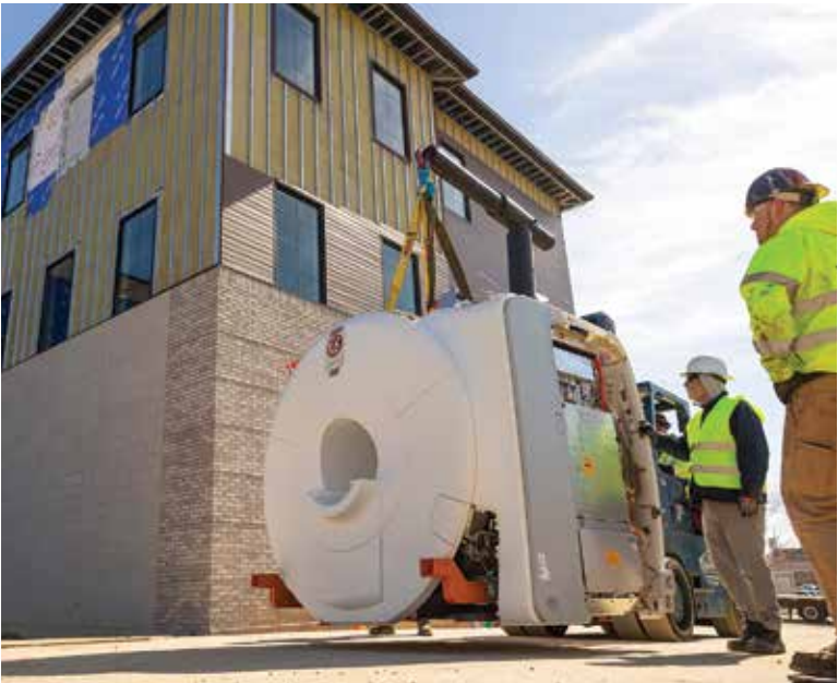
Workers prepare to deliver the MRI system to the basement of the Veldman Family Psychology Clinic. (Photo by Jon Hendricks)
