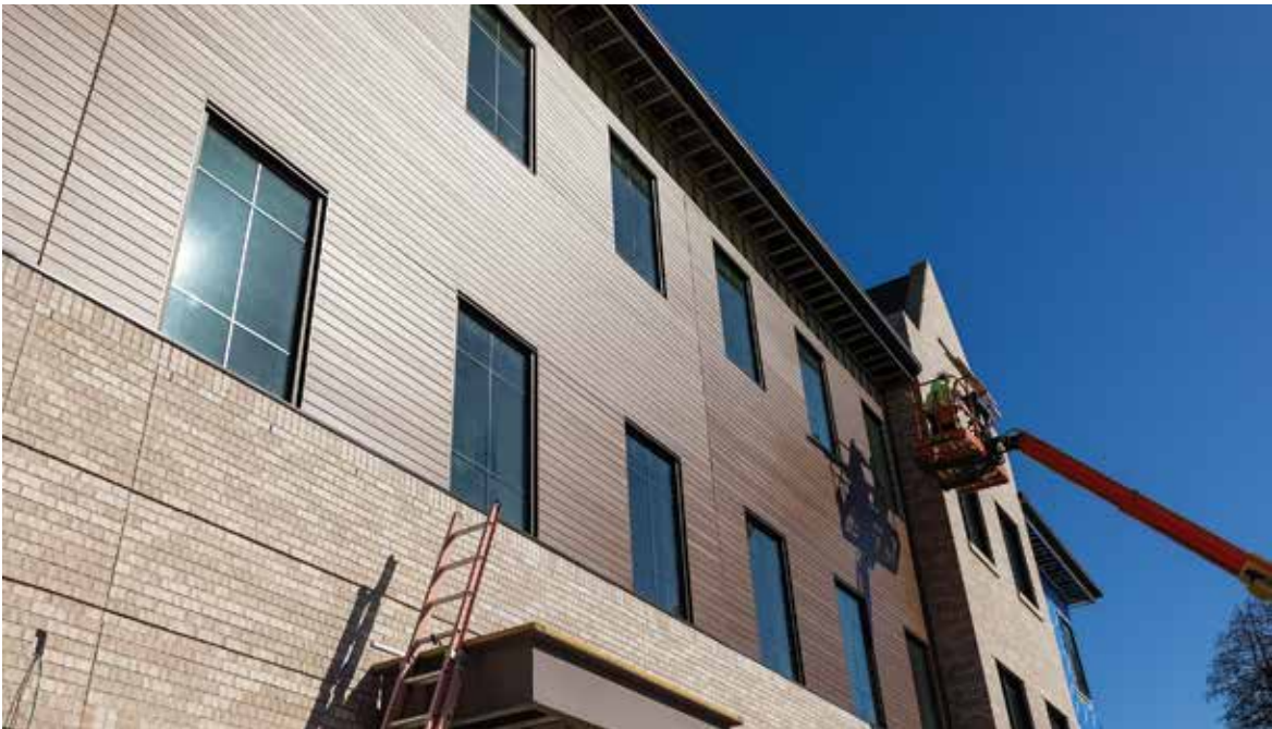
Work is being completed on the Veldman Family Psychology Clinic. (Photo by Jon Hendricks)
